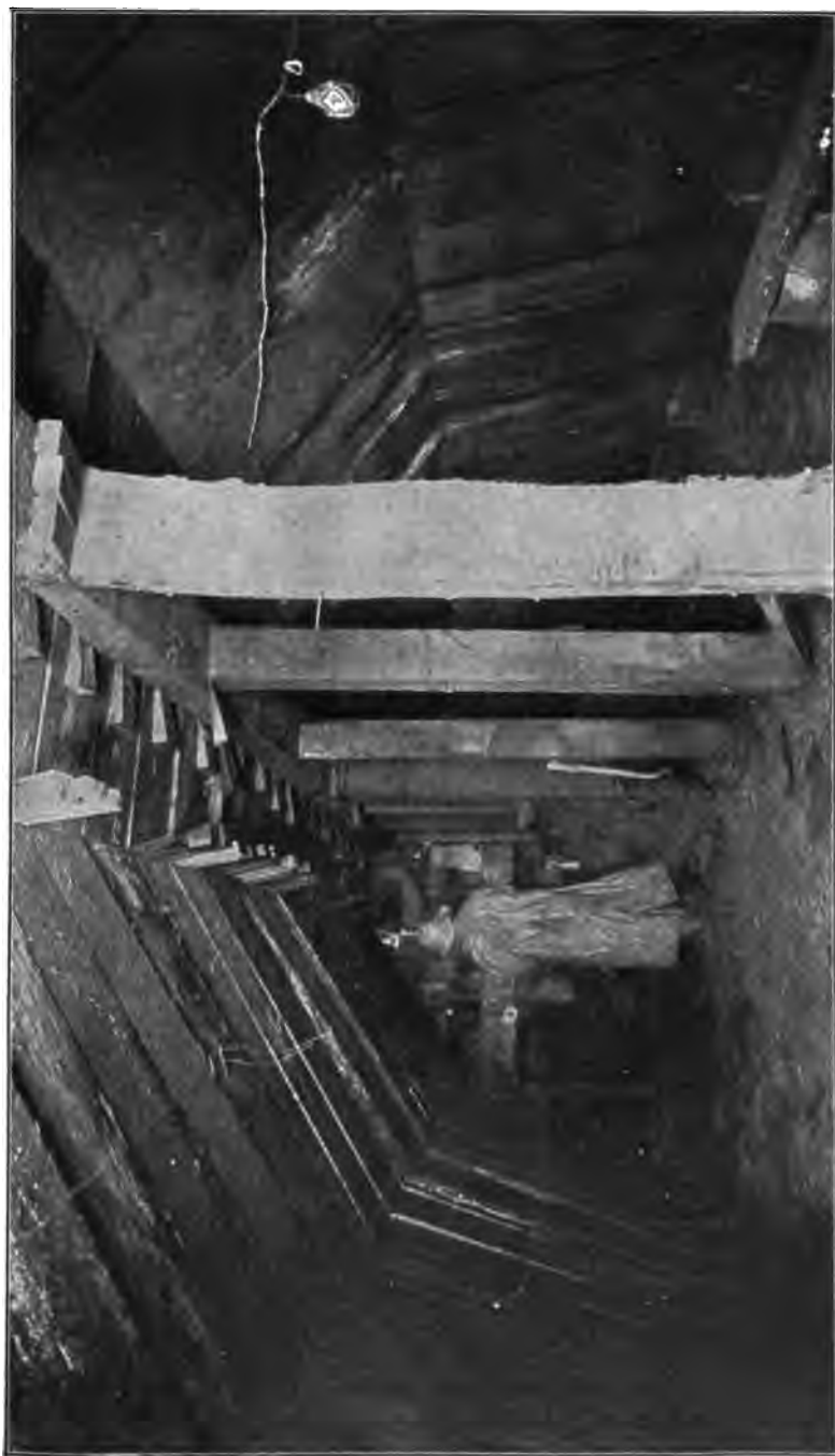
PLATE 187.—Contract 52. Eastview Tunnel. Heavy Timbering in Compressed Air.
